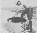
Luis J. Maduro, an Assistant Operator in the Clean Oils/Crude Area hand tapes a tank to compare with "Varec" gauge reading.
